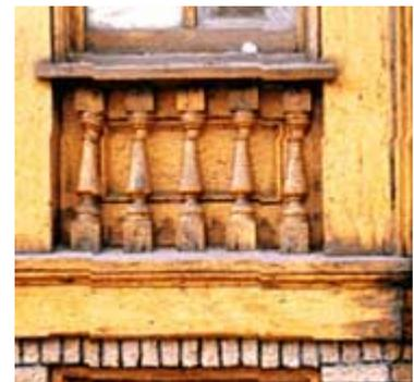
When the protective and decorative paint finish was removed and an inappropriate clear finish applied, the exterior character of the building was altered. Photo: NPS files.
